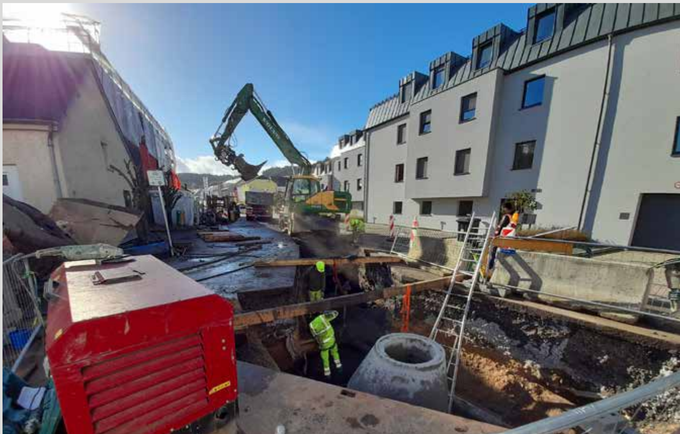
Chantier Goussel – (Foto: Paul Provost)
