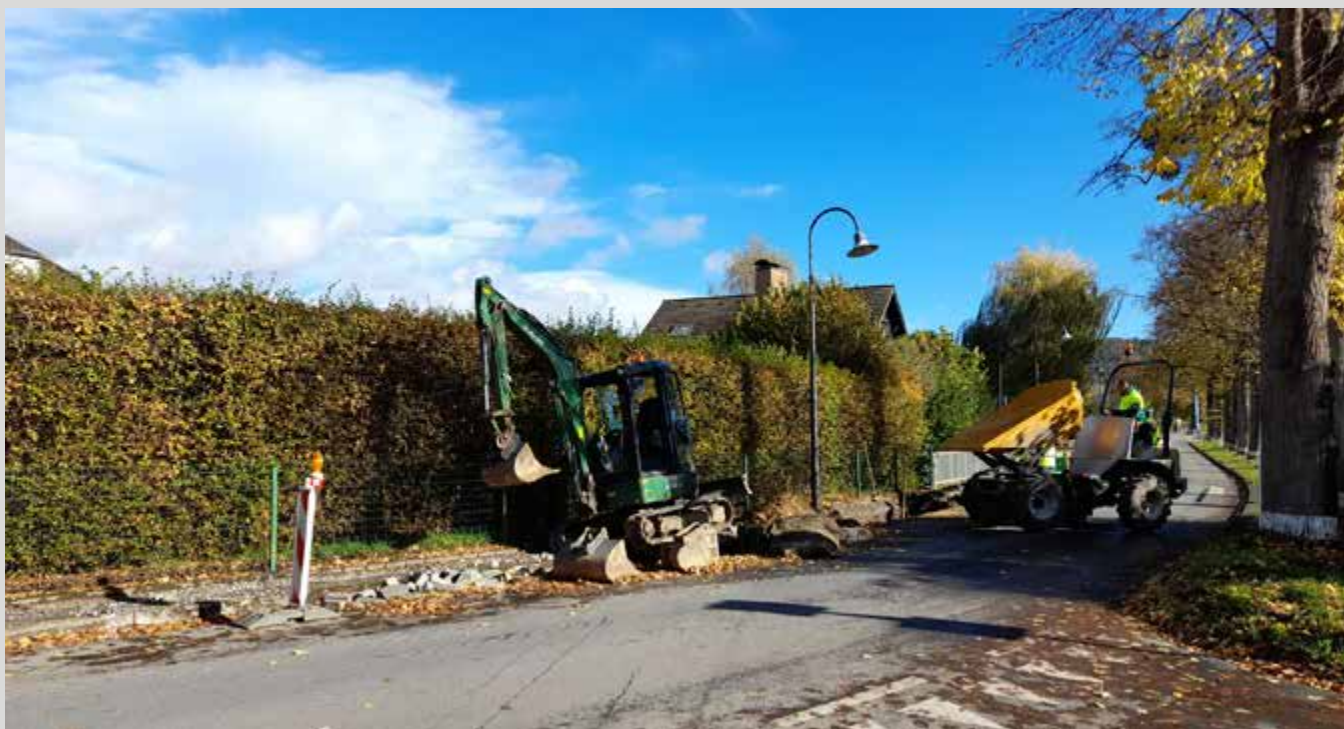
Chantier Goussel – (Foto: Paul Provost)
