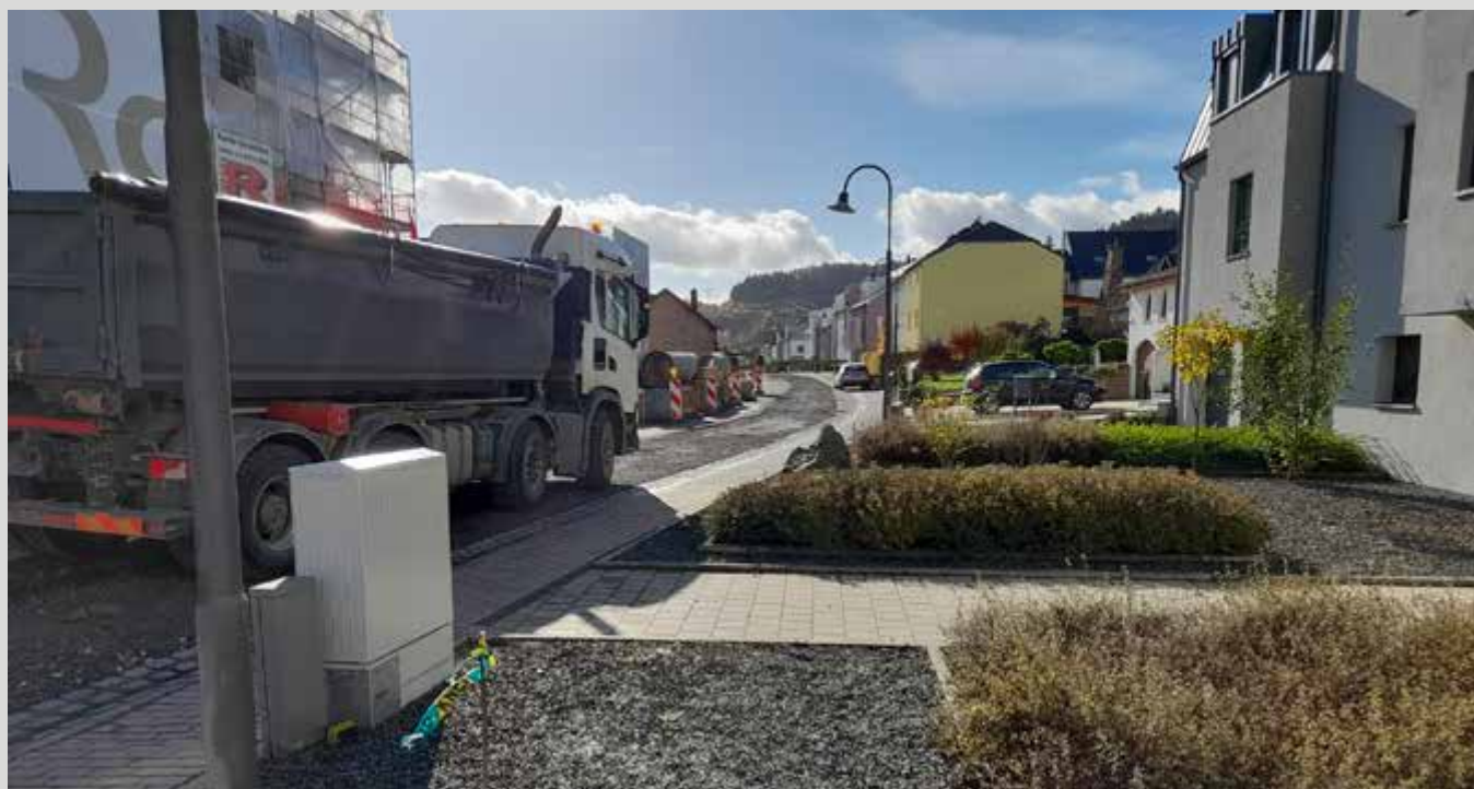
Chantier Goussel - (Foto: Paul Provost)
