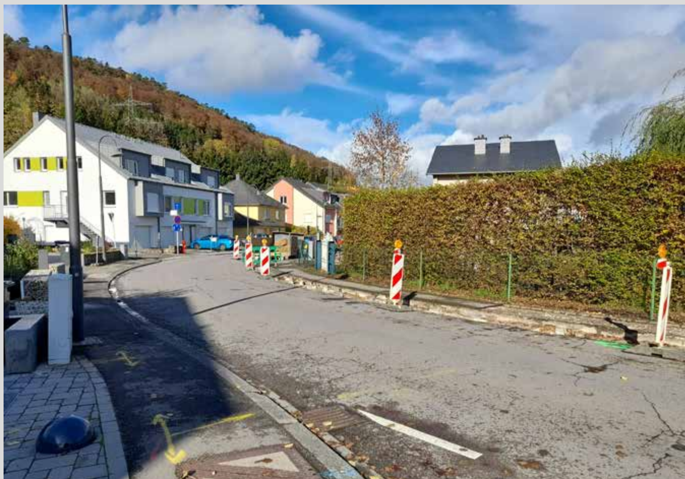
Chantier Goussel – (Foto: Paul Provost)
